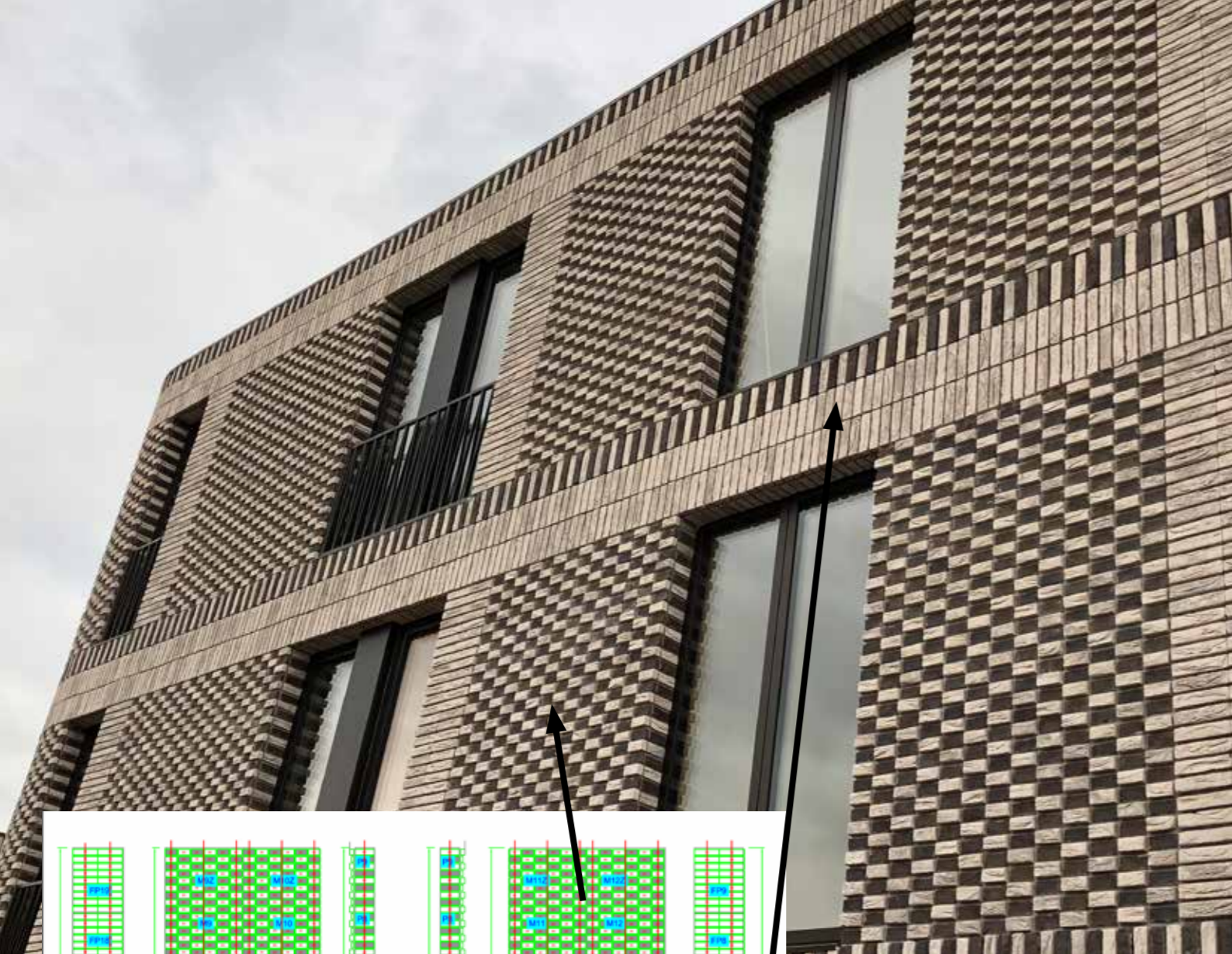
Typical Soldier Course with Stretcher Panel set out.
