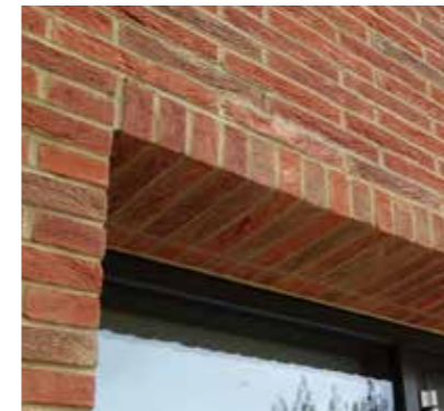
Header Bond Lintel Unit
